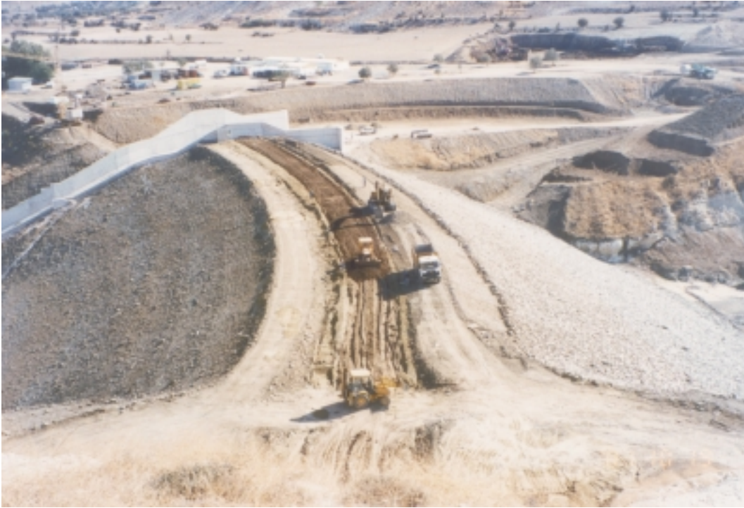
Tamasos (Under Construction)
